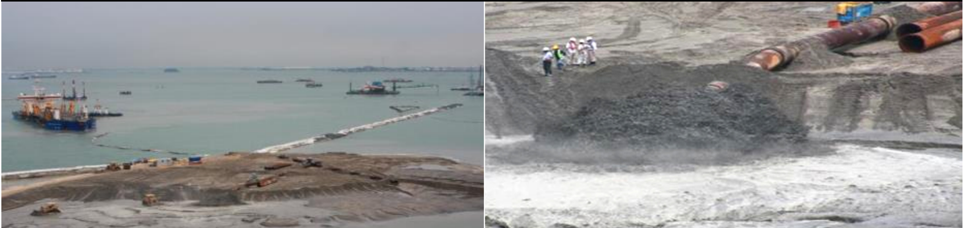
Trailer Suction Hopper Dredger (TSHD) connected via Land Pipeline
